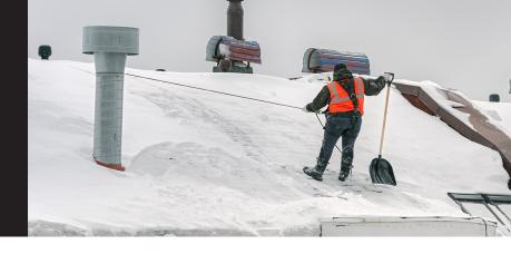
MSI is aware of snow loads on school buildings starting to show strains of such things as beams cracking, potential leakage from the melt etc. We are advising all Divisions to ensure that roofs are cleared of snow to help mitigate potential issues such as collapse or water infiltration before the melting season begins.
